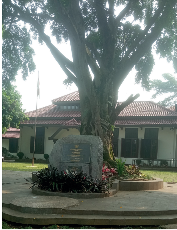
Fig. 3: Indonesia Menggugat building from the front.
